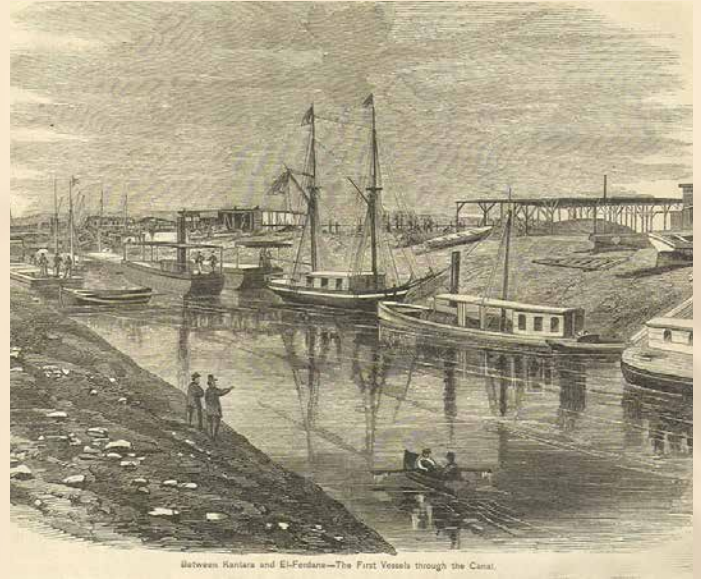
Between Kanara and El-Fendana—The First Vessels through the Canal.
